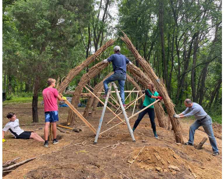
YAROUB AL-OBAIDI, FAR RIGHT, AND SARAH KAVAGE, 2ND FROM RIGHT, ESTABLISH THE FOUNDATION WITH PARABOLIC ARCHES OF BOUND REEDS.
