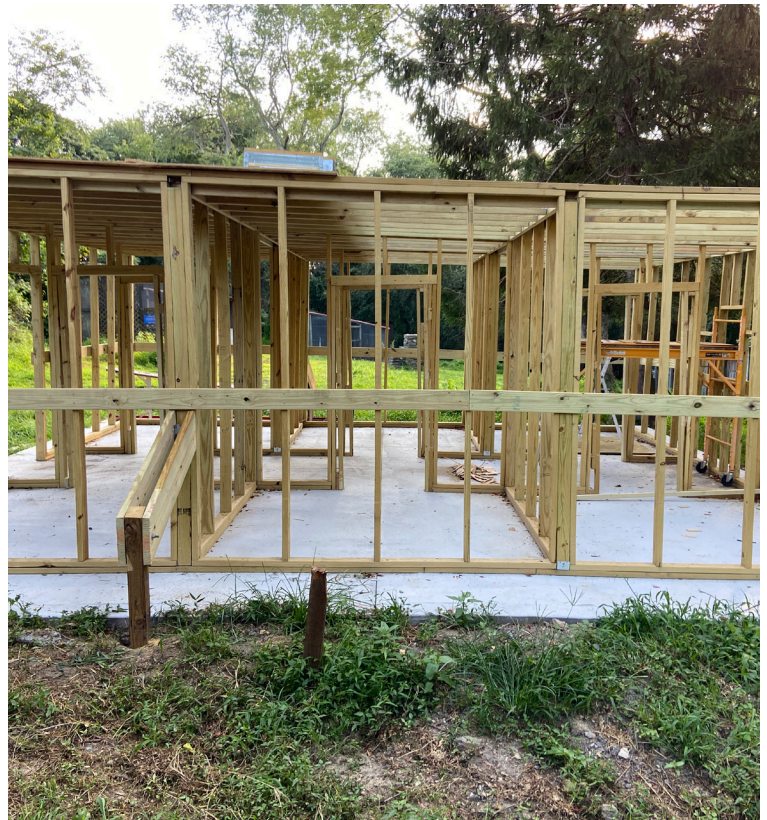
ABOVE: FRAMING FOR SQUIRREL ENCLOSURE
